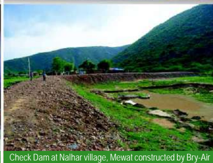
Check Dam at Nalhar village, Mewat constructed by Bry-Air
